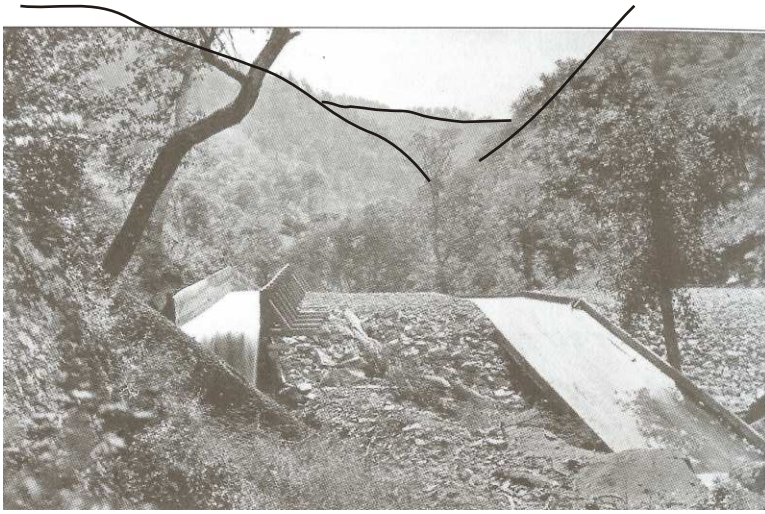
Huachuca Water Company Dam in Miller Canyon.
